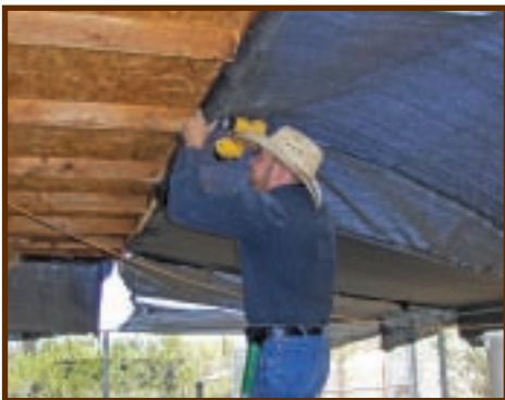
Jonny Repairing Summer Shade On The Pens' Roof
